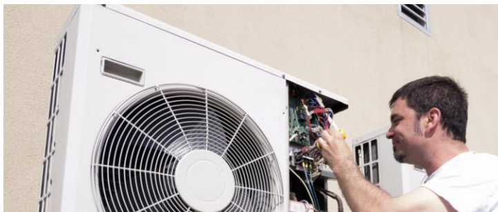
Figure 11: The Heat Pump Store staff installing in Portland, OR.
