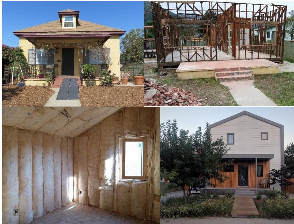
Figure 31: The Perlita Passive House: the original house was stripped to the studs, re-insulated, tested and made into an LA modern masterpiece of efficiency. 76
